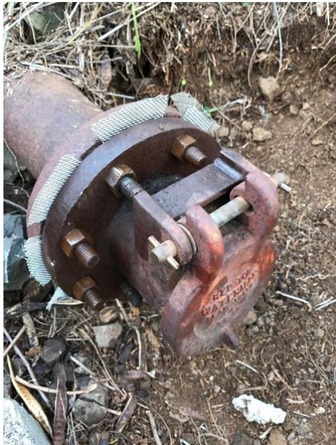
Photo of screen installed between the flange.
