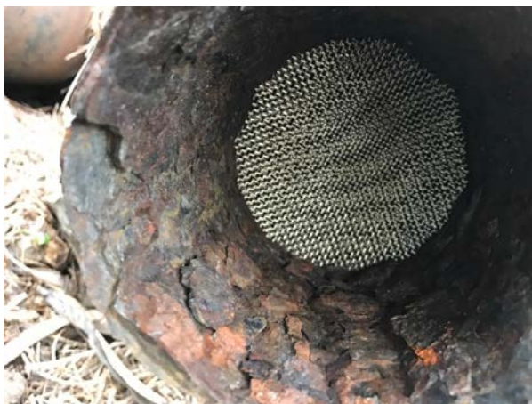
Picture of screen inside pipe.
