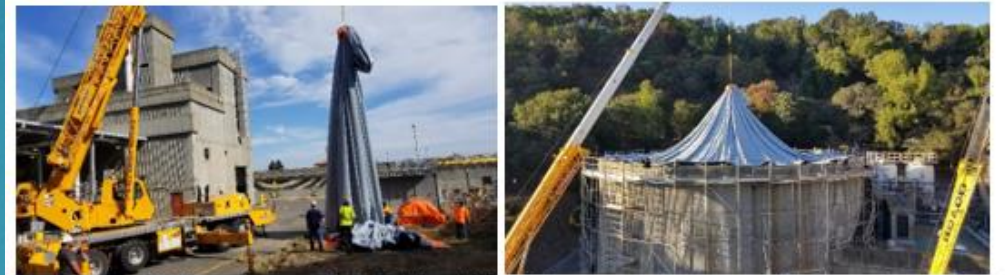
Figure 6: GrayWolf was back onsite in October to install the new membrane cover (inner membrane shown).
