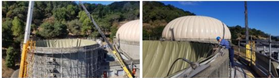
Figure 2: GrayWolf removed the membrane cover in August. A crane was used to remove the cover, and a lift was used to lower the contractor in to remove the cable hub and level sensor.
