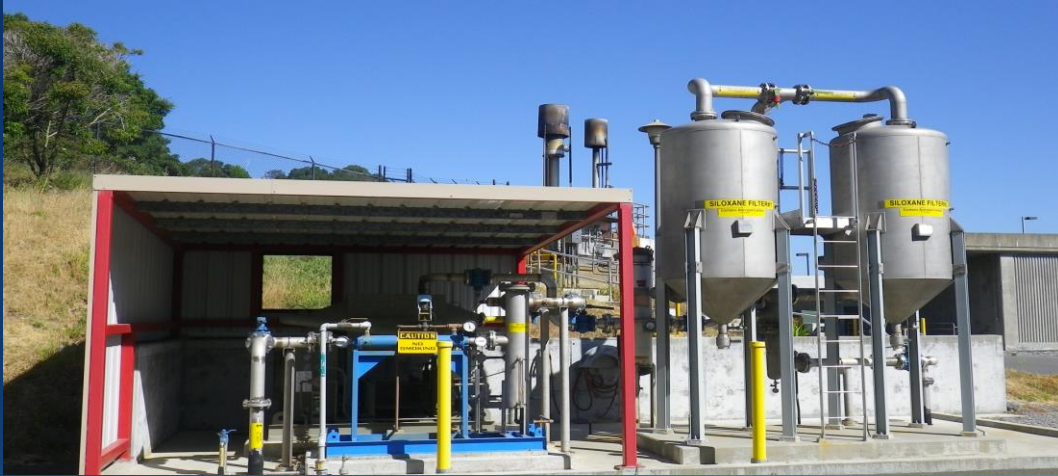
Biogas - moisture and siloxane removal
