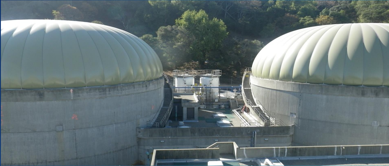
Anaerobic digesters with membrane covers
