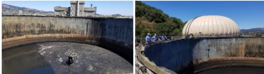
Figure 3: After the cover was removed, Operations began draining the digester.
