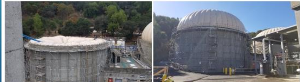
Figure 8: Inflating the outer membrane (left) and completed installation (right).
