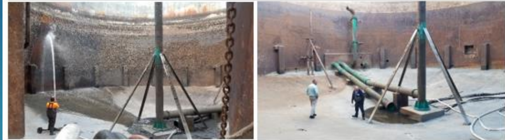
Figure 5: Wastewater Solids Management pressure washed the inside of Digester 2 and staff inspected it.
