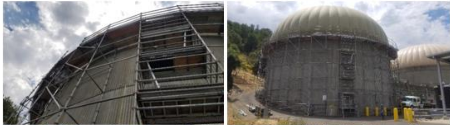
Figure 1: Scaffolding was installed around the 80-ft diameter digester (37.5-ft tall) in July to provide access for the contractor (GrayWolf) to remove and install the cover.
