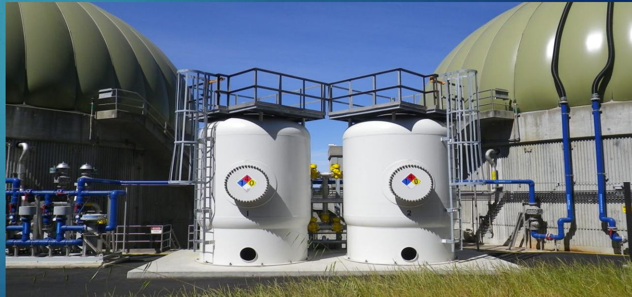
Biogas H 2 S Removal
