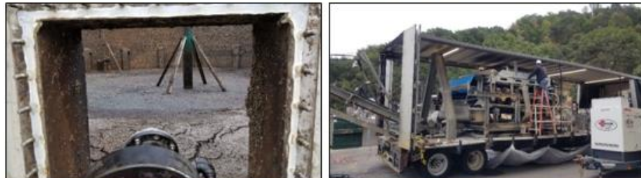
Figure 4: Staff contracted Wastewater Solids Management in September to clean and remove the sludge, grit and debris that was accumulated inside the digester. A belt filter press was onsite to dewater the solids.
