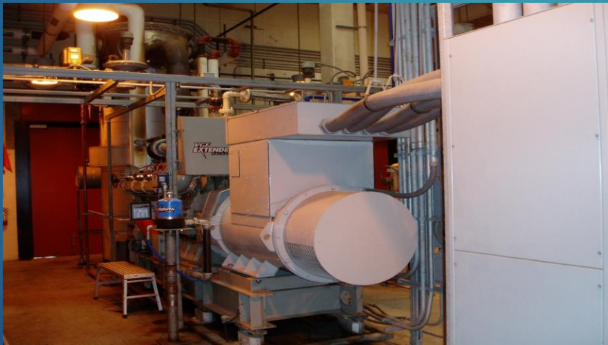
Back-up 750 kW Cogen System (Waukesha)
