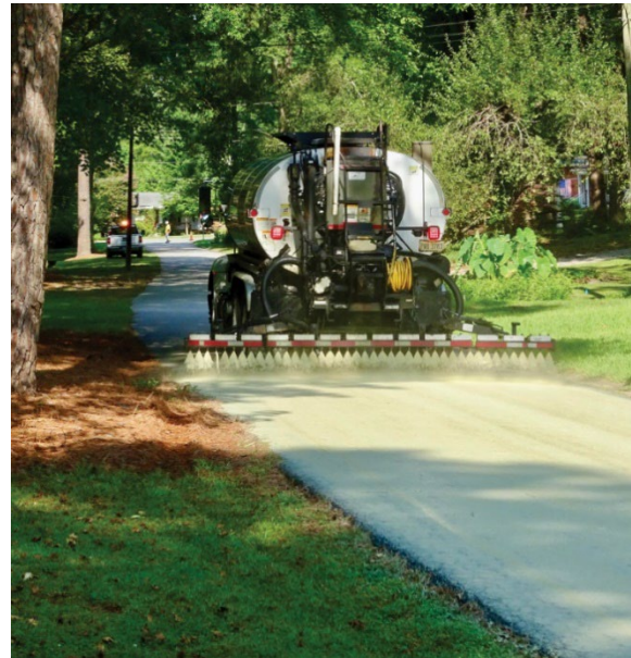
Picture 1: Photocatalytic pavement treatment in Raleigh, NC
