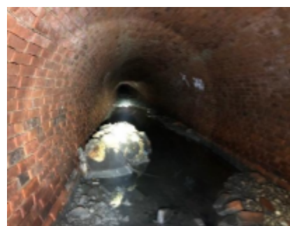
Example of Failing Sewer in a West Louisville LIDAC
