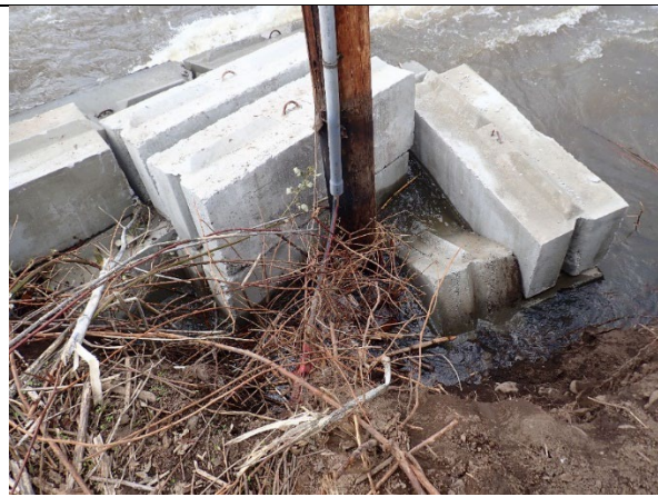
Calkins Property Damage showing power pole that was nearly washed out on April 16, 2019. The power line did not wash out due to emergency managers places structural support on the pole base, but the utility company had to move the line.
